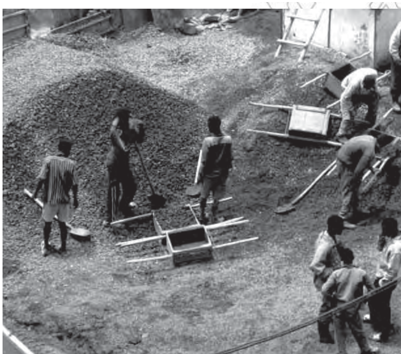
A group of blue collar workers on a building site
